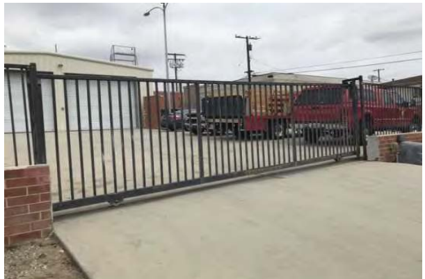
12 VEHICLE CONTROL GATE
