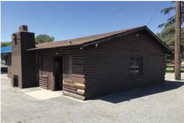
39 STORAGE BUILDING RIGHT/REAR ELEVATION
