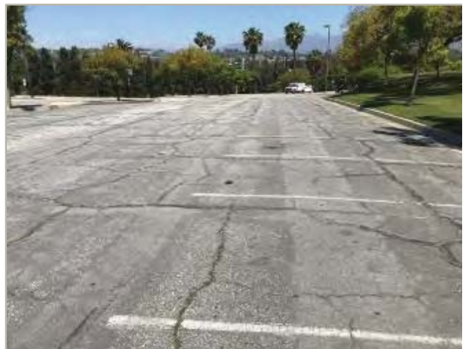
Exterior path of travel
