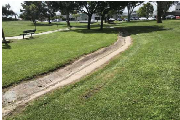
10 DRAINAGE SWALE
