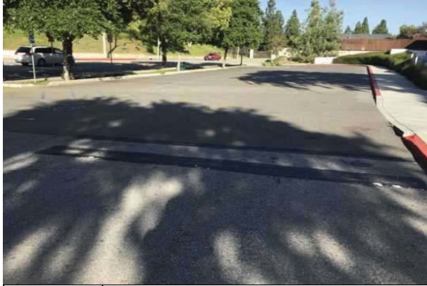
31 ASPHALT PARKING LOT PAVEMENT
