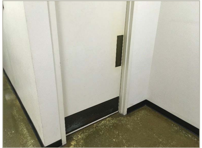
Interior accessible doorway
