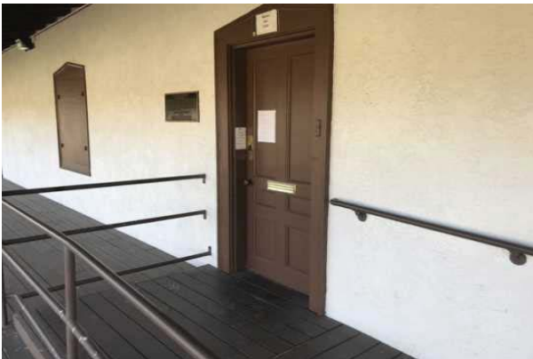
35 MAIN EXTERIOR DOOR
