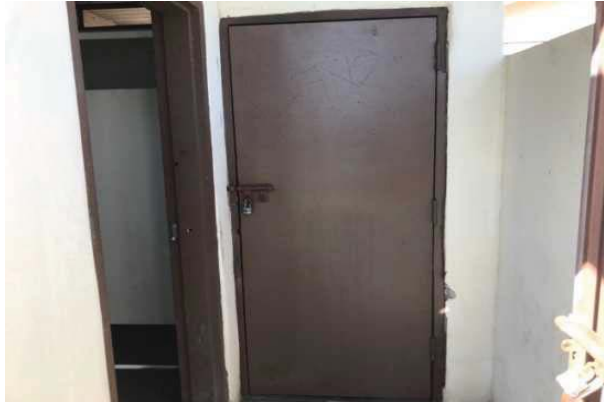
38 RESTROOM INTERIOR DOOR
