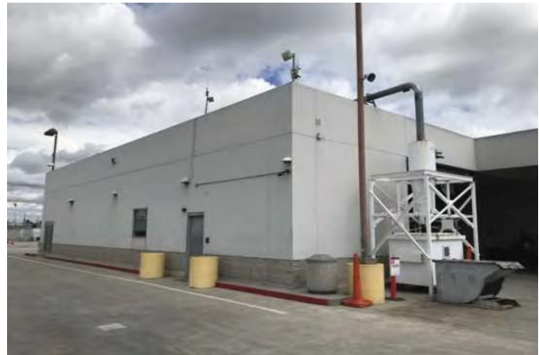
16 FUEL BUILDING/BUS WASH
