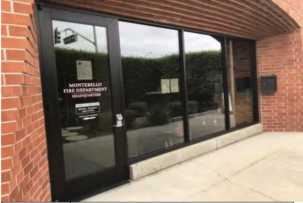
19 MAIN EXTERIOR DOOR
