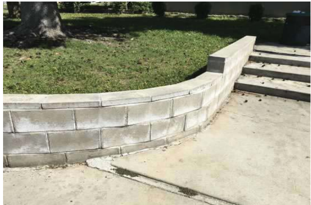
10 CONCRETE SIDEWALK, STAIRS, AND RETAINING WALL
