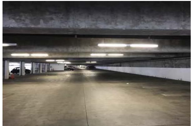
22 PARKING STRUCTURE LOWER LEVEL
