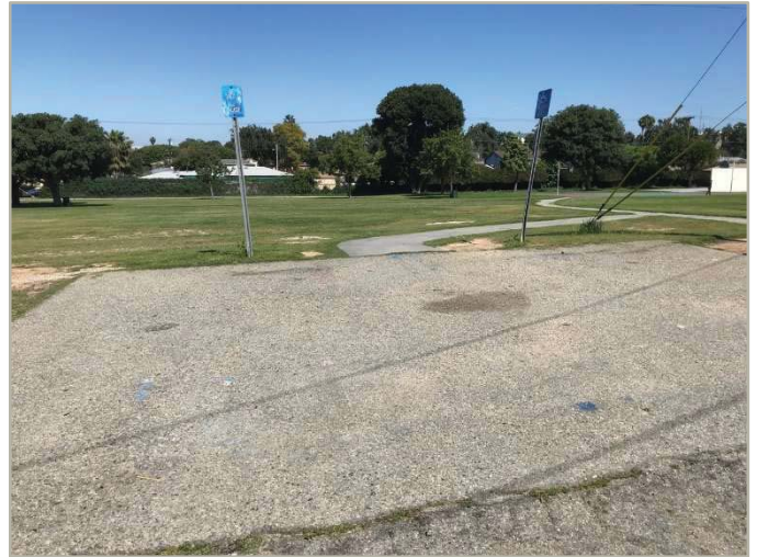
Exterior Route Access
