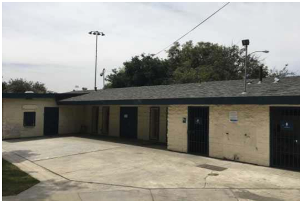
5 RESTROOM - FIELD 1, SOUTH
