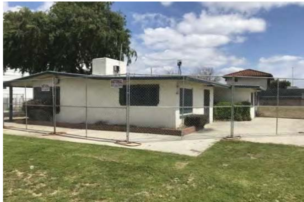
52 PARK RANGERS BUILDING EXTERIOR
