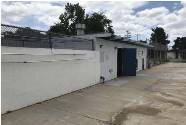
41 POOL EQUIPMENT BUILDING
