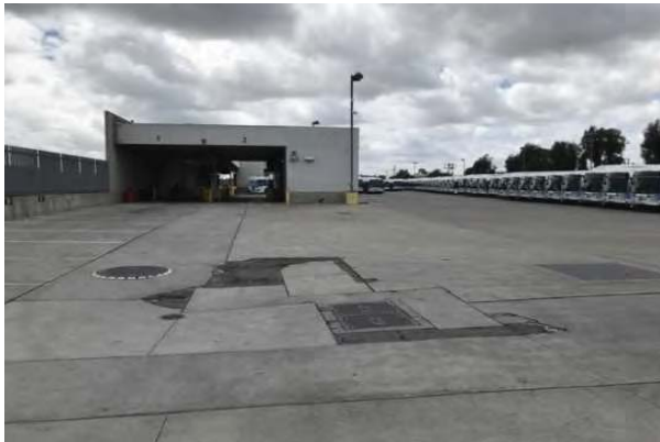
15 FUEL BUILDING/BUS WASH
