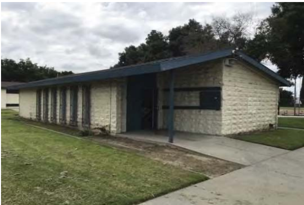
35 CONCESSION BUILDING - FRONT/RIGHT ELEVATIONS
