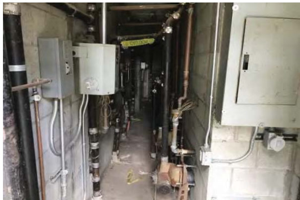
34 RESTROOMS BUILDING PLUMBING
