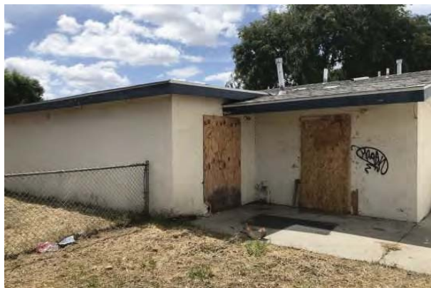
54 SCOUT HOUSE BUILDING EXTERIOR
