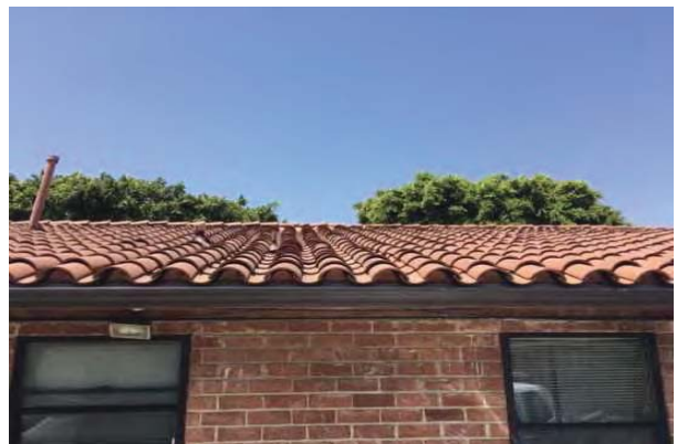
18 CLAY TILE ROOF
