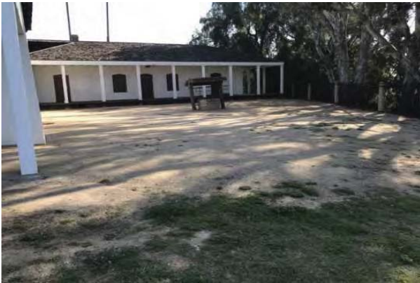
15 ERODED LANDSCAPING AREAS
