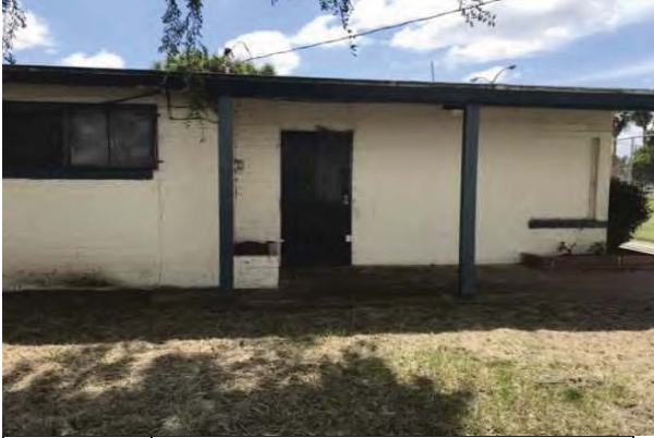
49 PARK RANGERS BUILDING EXTERIOR
