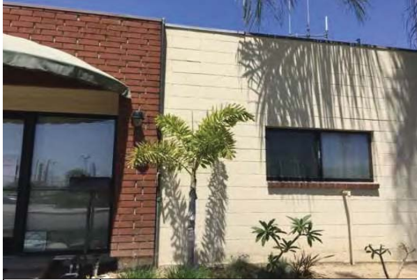
13 BRICK, CMU, AND ALUMINUM WINDOW FAÇADE
