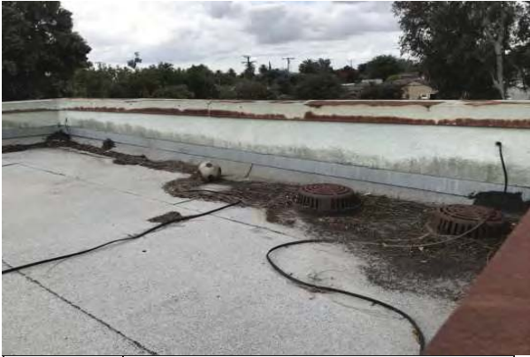
37 COMMUNITY BUILDING ROOF
