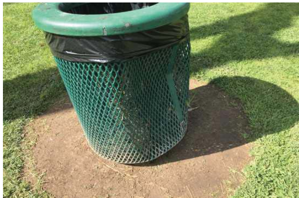
30 DAMAGED PARK TRASH RECEPTACLE
