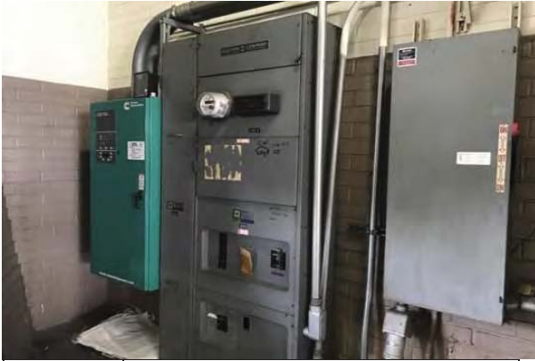
31 BUILDING/MAIN SWITCHBOARD
