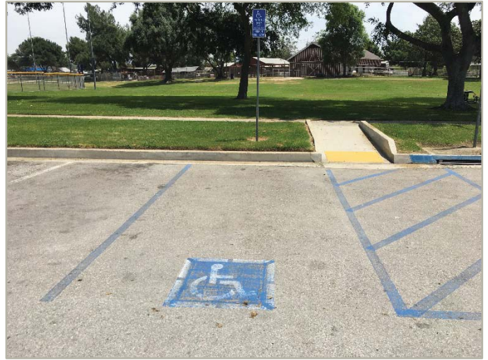
Van accessible parking stall
