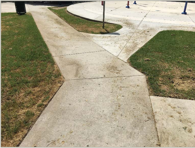
Exterior path of travel
