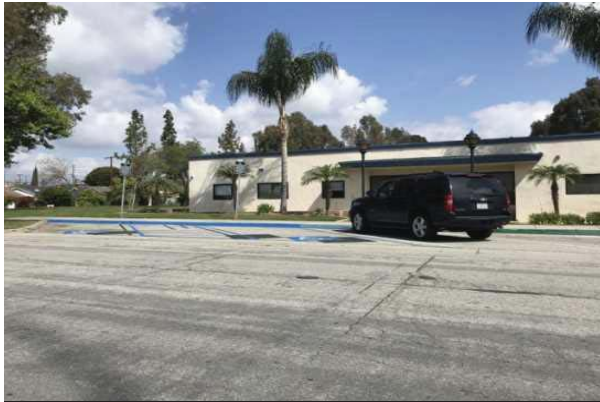
7 ADA PARKING ALONG VICTORIA
