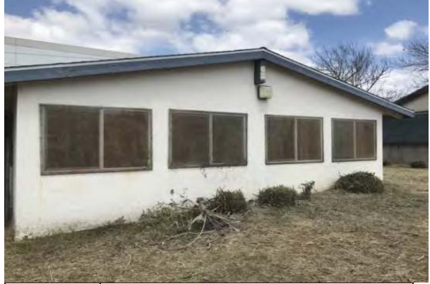
56 SCOUT HOUSE BUILDING EXTERIOR
