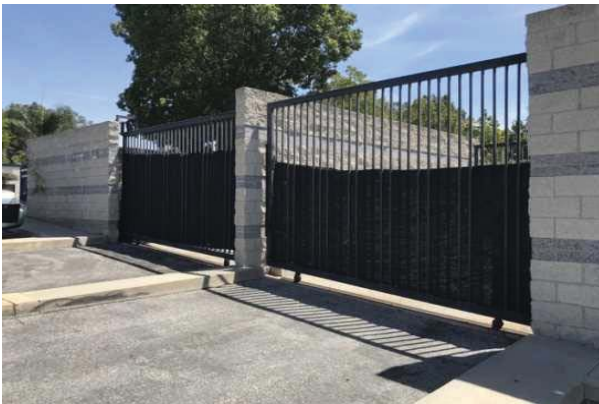
17 VEHICLE CONTROL GATE
