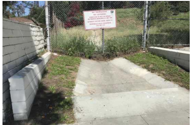
10 DRAINAGE SWALE
