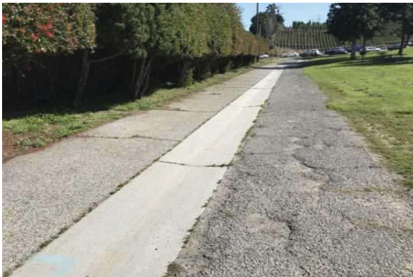
11 DRAINAGE CONCRETE SWALE
