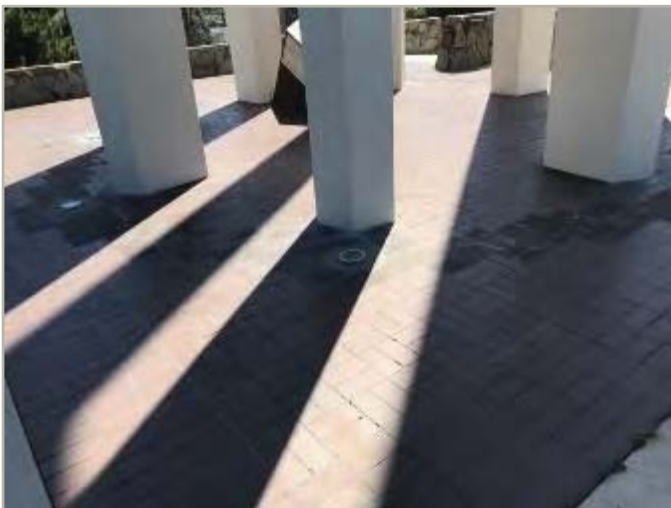
Interior path of travel
