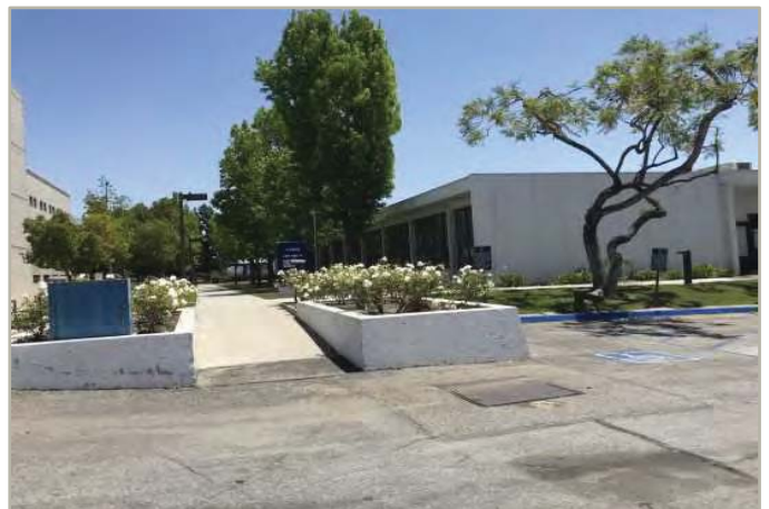
Accessible parking with ramp
