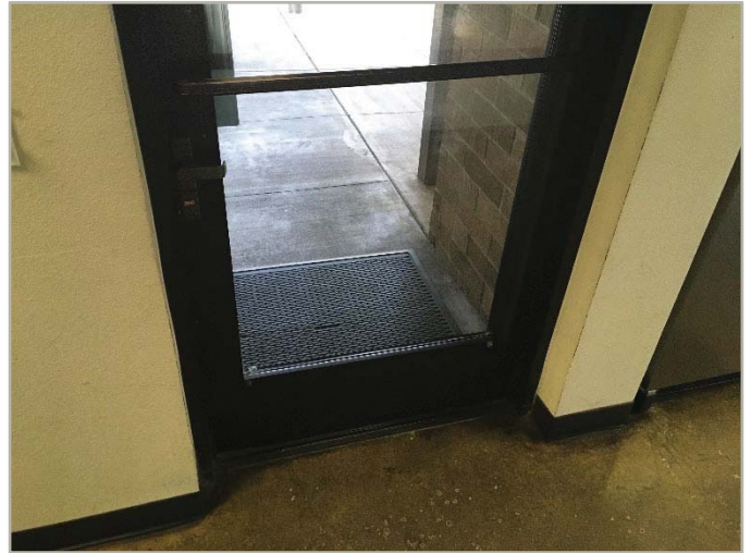
Alternative building entrance
