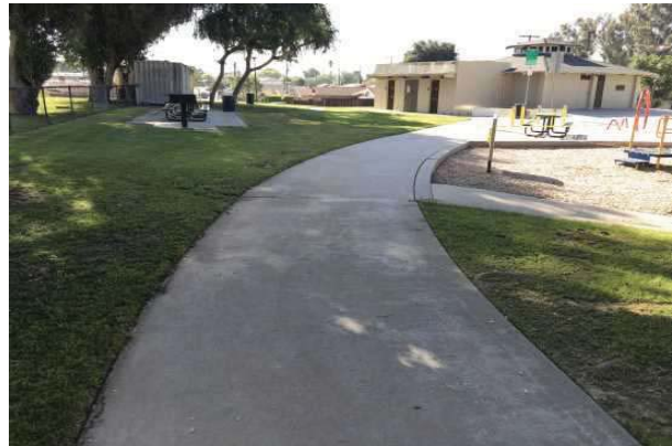
28 PEDESTRIAN CONCRETE PAVEMENT
