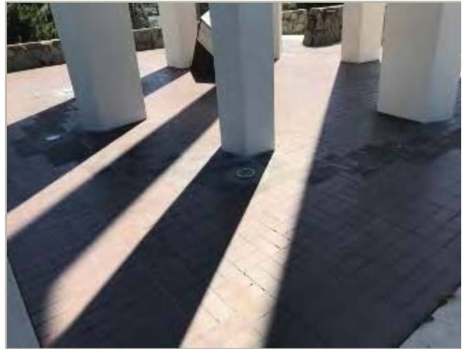
Interior path of travel
