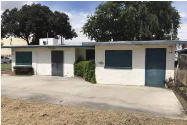
51 PARK RANGERS BUILDING EXTERIOR
