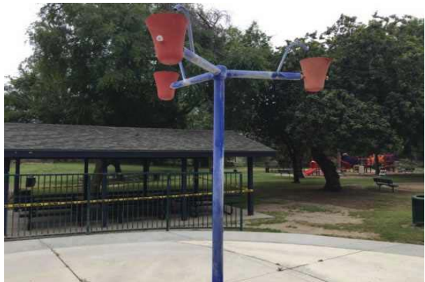
48 AQUATIC PLAY STRUCTURE
