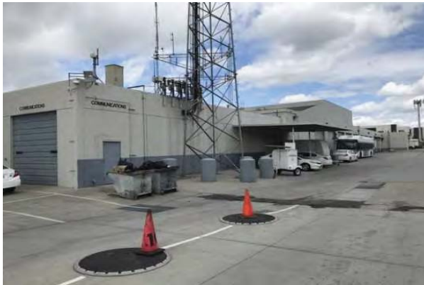
9 COMMUNICATION BUILDING EXTERIOR
