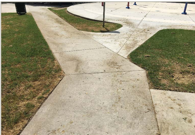
Exterior path of travel
