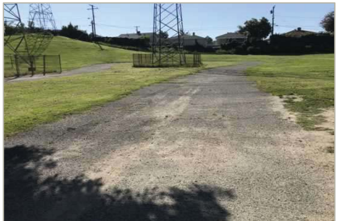
Exterior path of travel
