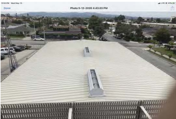
17 VEHICLE HANGER ROOF
