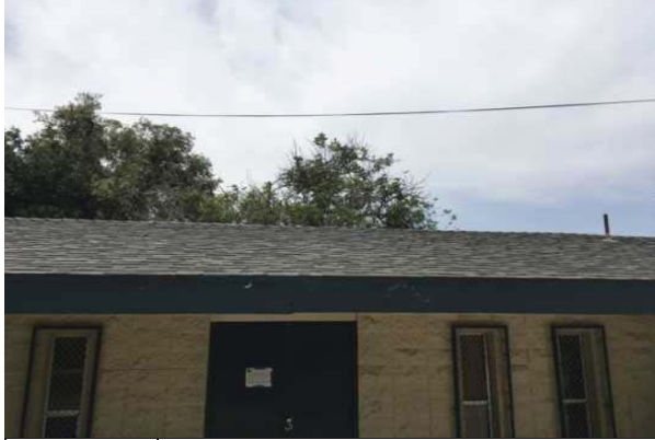
13 ASPHALT SHINGLE ROOF
