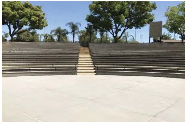
28 BANDSHELL BUILDING STAGE
