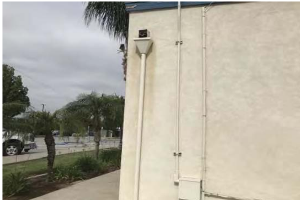
16 GUTTERS AND DOWNSPOUTS
