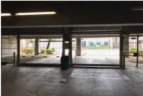
21 PARKING STRUCTURE LOWER LEVEL GATES
