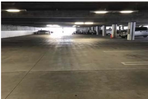
23 PARKING STRUCTURE LOWER LEVEL
