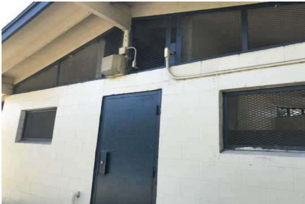
39 UTILITY EXTERIOR DOOR
