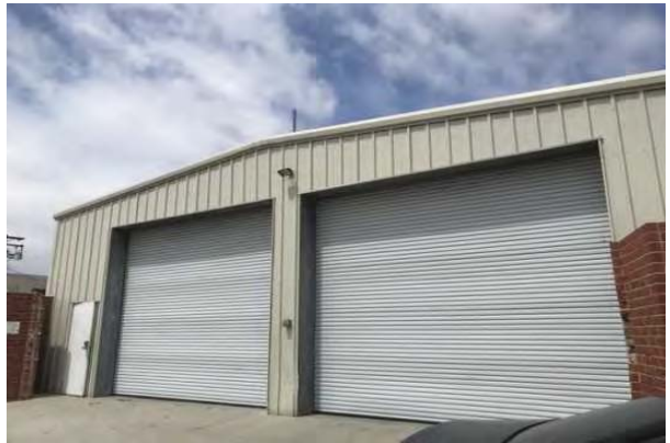
22 REAR OVERHEAD DOOR
