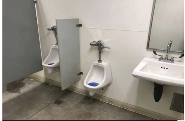
50 COMMUNITY CENTER RESTROOM
