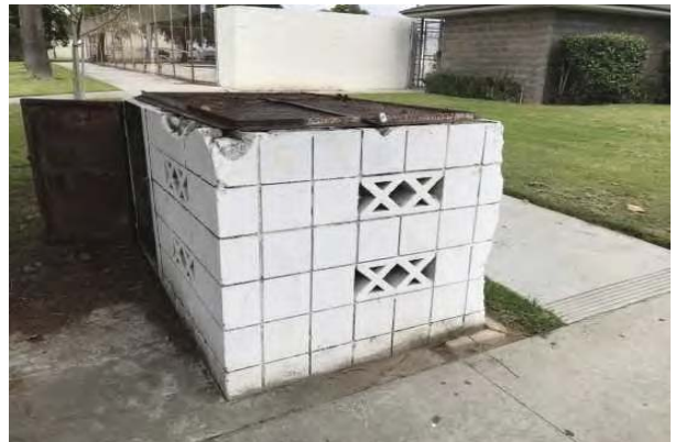
24 IRRIGATION PUMP HOUSE
