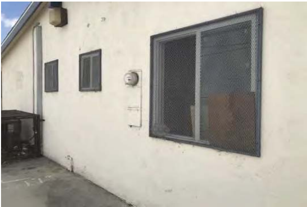
57 SCOUT HOUSE BUILDING EXTERIOR
