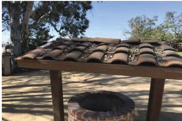
34 FIRE PIT ROOF
