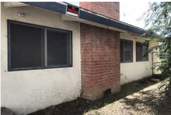
53 SCOUT HOUSE BUILDING EXTERIOR
