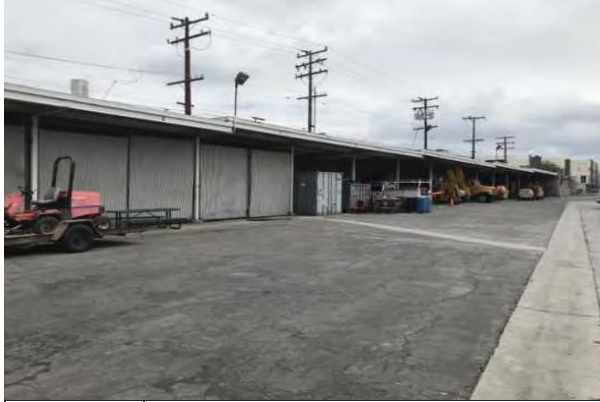
13 STORAGE SHED STRUCTURE
