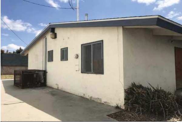
55 SCOUT HOUSE BUILDING EXTERIOR
