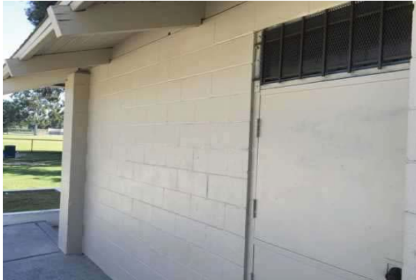
7 EXTERIOR PAINTED CMU WALL
