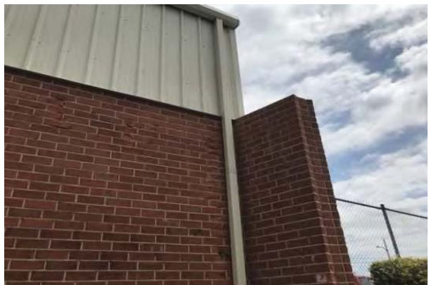
18 GUTTERS AND DOWNSPOUTS
