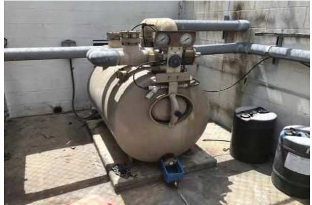
44 SWIMMING POOL FILTRATION SYSTEM
