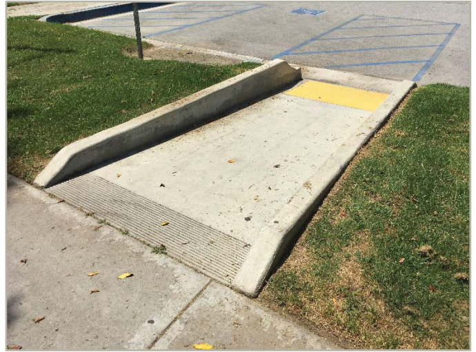
Exterior path of travel
