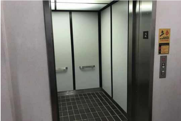
25 ELEVATOR CAB FINISHES
