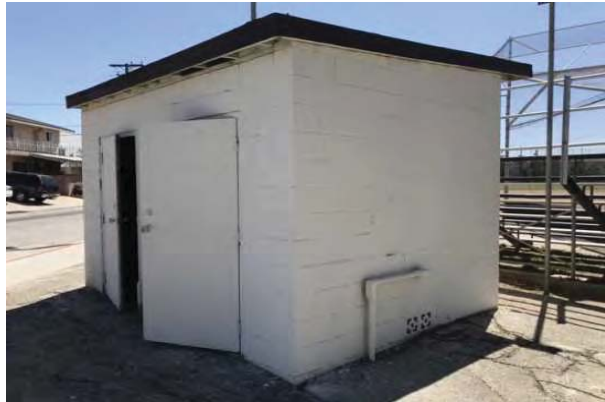
48 SOFTBALL FIELD UTILITY BUILDING
