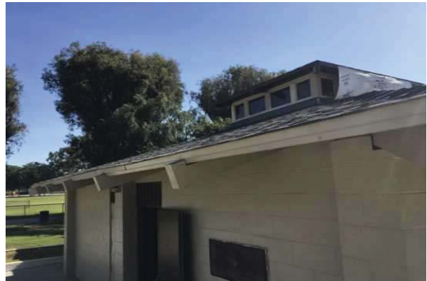
10 ASPHALT SHINGLES ROOF
