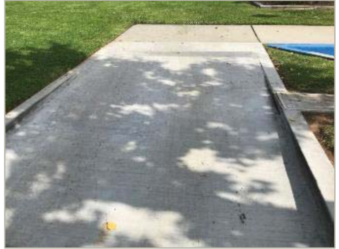
Accessible exterior path of travel
