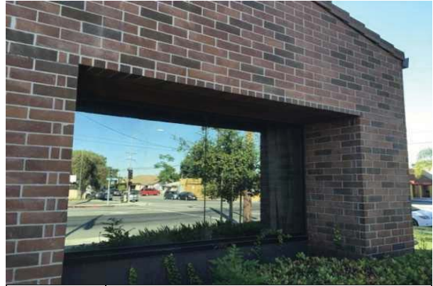
14 BRICK VENEER AND STOREFRONT WINDOW FAÇADE
