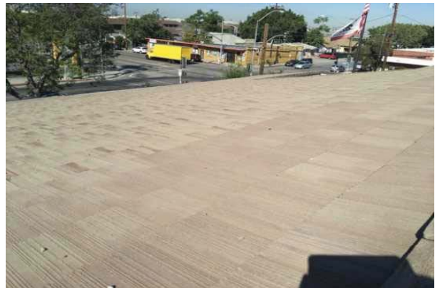
18 CONCRETE TILE ROOF
