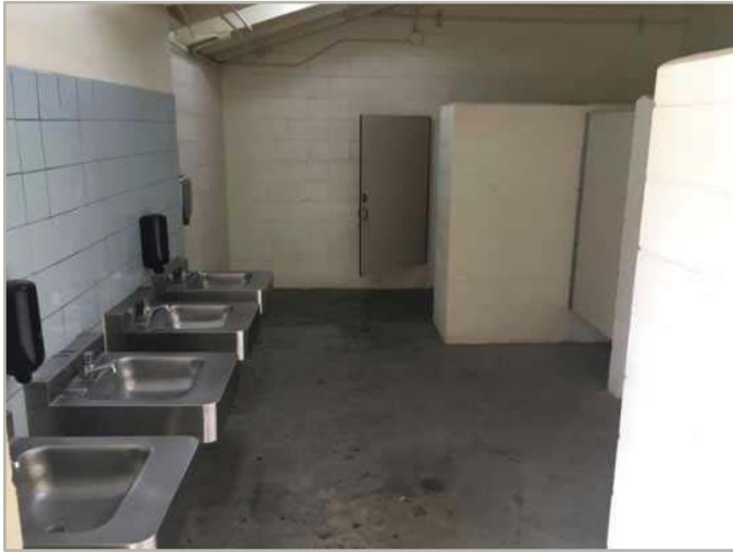
Rec center restroom
