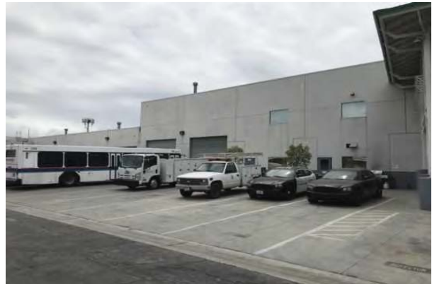
10 MAINTENANCE SHOP EXTERIOR
