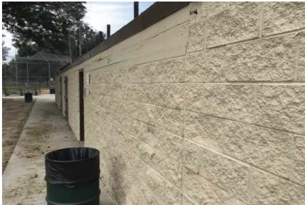
15 EXTERIOR PAINTED CMU WALL
