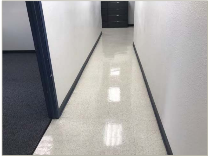
Interior path of travel
