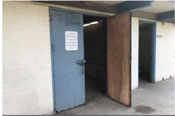
38 RESTROOM STORAGE ROOM EXTERIOR DOOR
