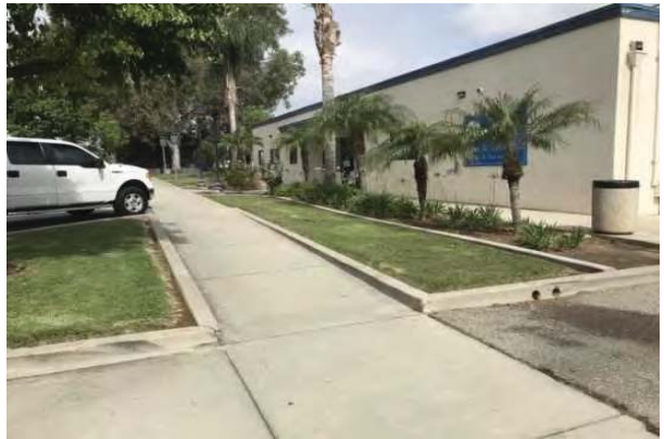
10 SIDEWALK AND EXTERIOR RAMP
