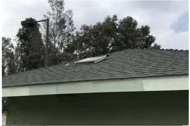
38 RESTROOM BUILDING ROOF
