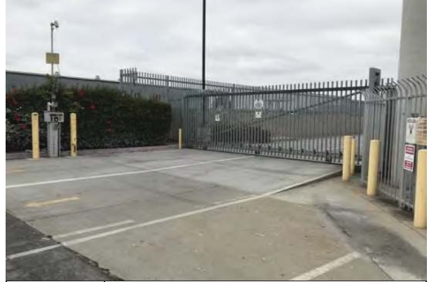
26 BUILDING 311 PARKING LOT- EAST ELEVATION GATE
