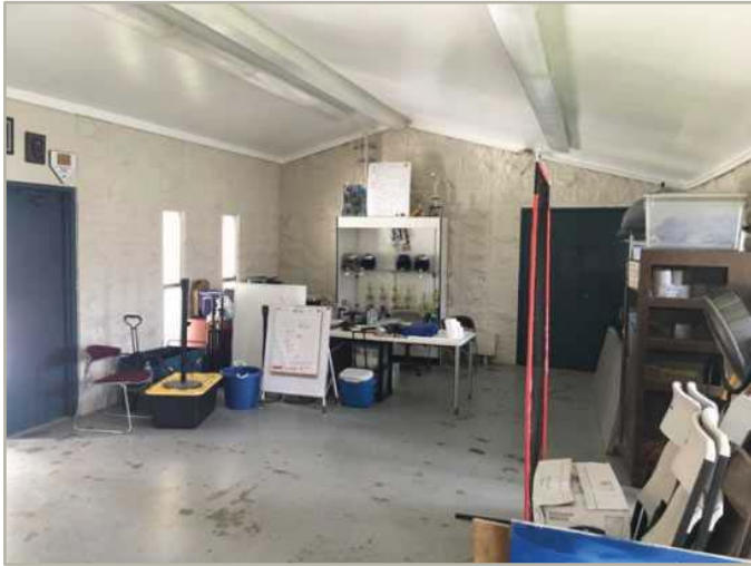
Field 1 south restroom building interior
