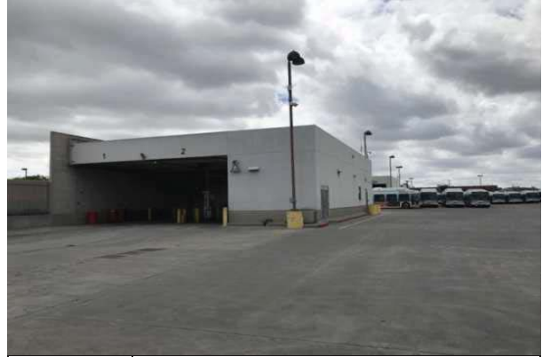
14 FUEL BUILDING/BUS WASH
