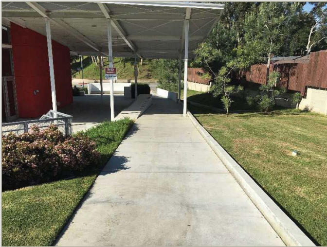
Park entrance ramp
