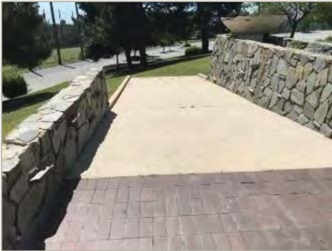
Building ramp entrance
