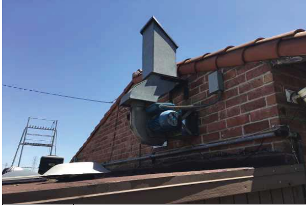
25 WALL MOUNTED VEHICLE EXHAUST FAN
