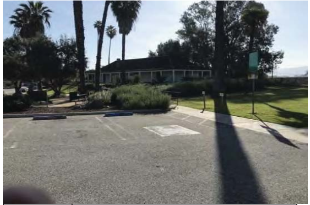
8 ADA, PARKING MISSING SIGN
