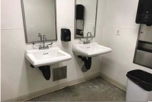
49 COMMUNITY CENTER RESTROOM
