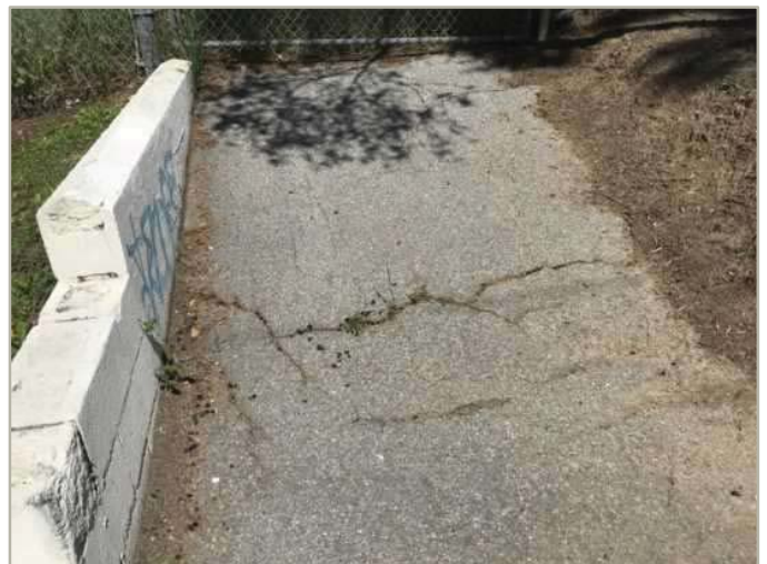
Service vehicle driveway
