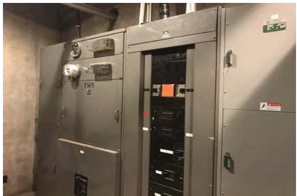
42 BUILDING/MAIN SWITCHBOARD
