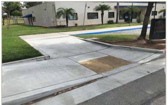
Exterior path of travel
