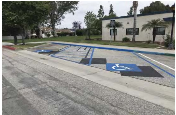
6 ADA STREET PARKING LOTS
