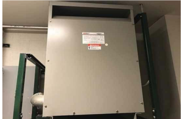
38 SECONDARY TRANSFORMER
