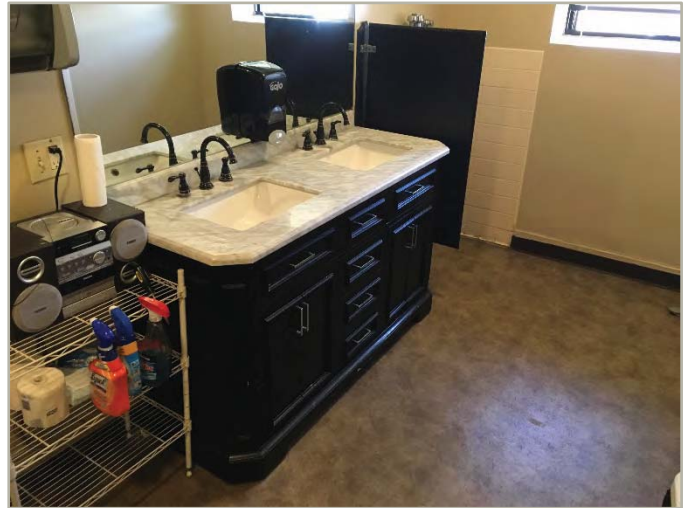
Inaccessible restroom accommodations
