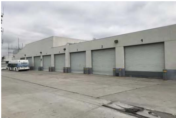
11 MAINTENANCE SHOP EXTERIOR
