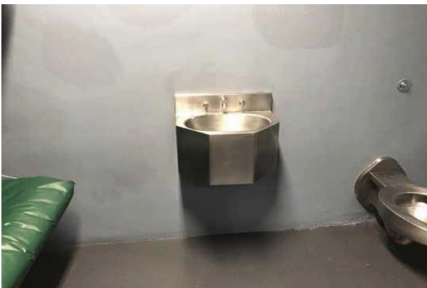
65 HOLDING CELL SINK AND TOILET
