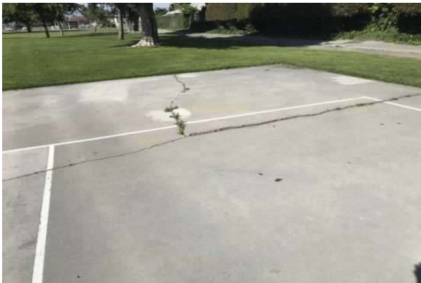
29 UNEVEN PEDESTRIAN PAVEMENT SIDEWALK
