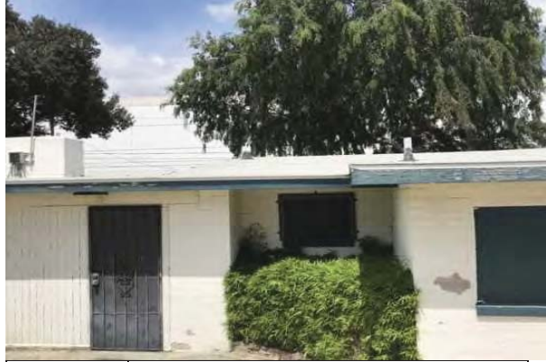
50 PARK RANGERS BUILDING EXTERIOR
