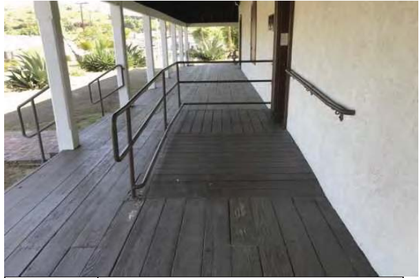
20 RAMP AT MAIN DOOR ENTRANCE
