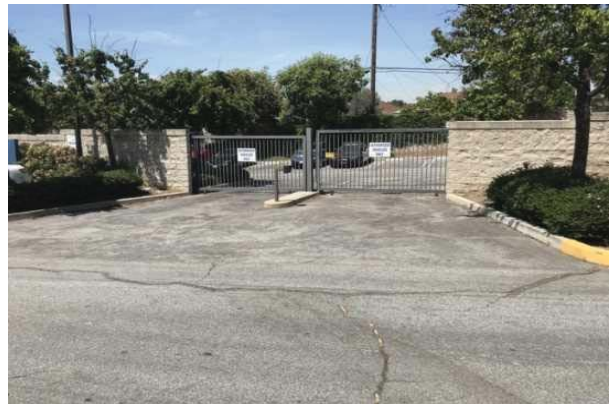
18 VEHICLE CONTROL GATE
