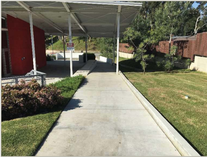
Park entrance ramp
