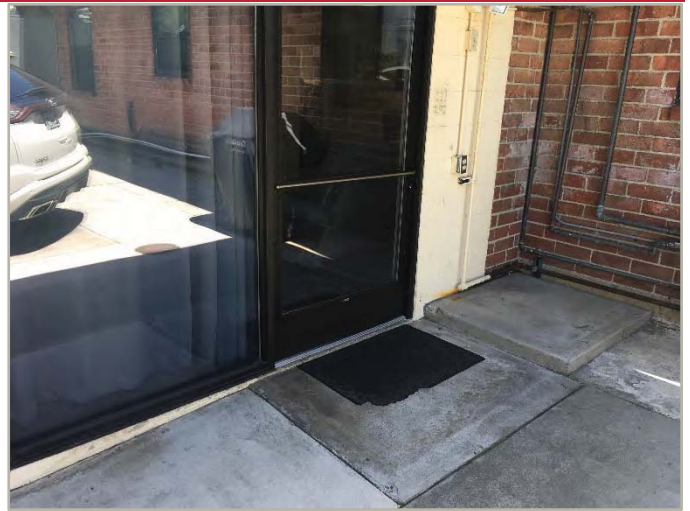
Alternative building entrance
