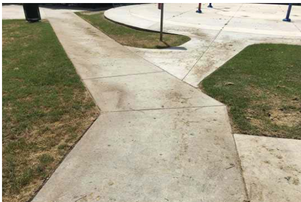
41 PEDESTRIAN CONCRETE PAVEMENT
