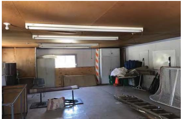
40 STORAGE BUILDING INTERIOR
