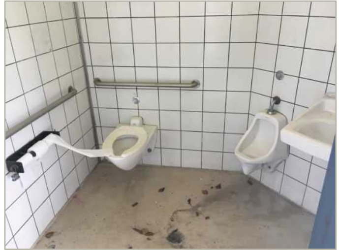
Field 1 north restroom building restroom
